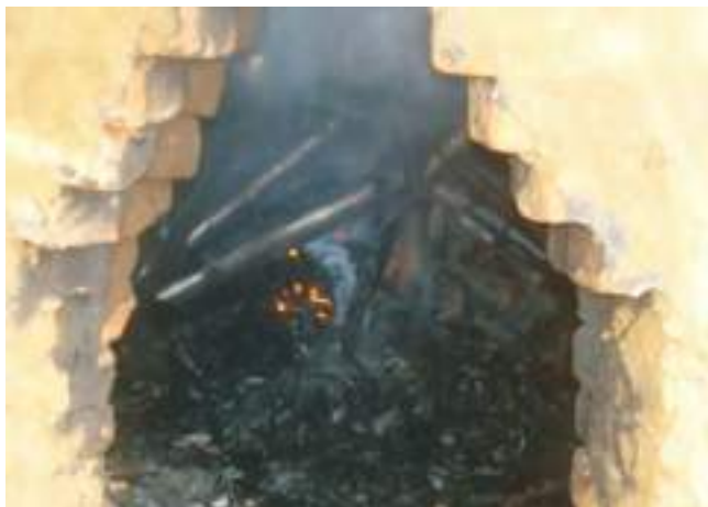
On Opening the Brick Kiln
