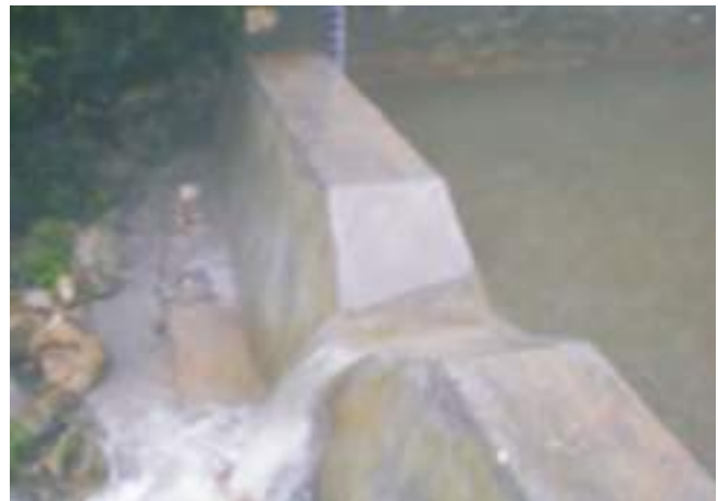
Weir at Site
