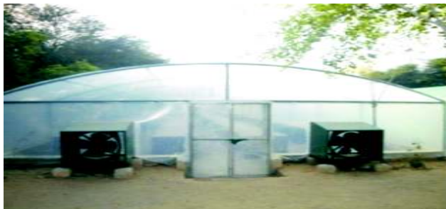
Renovated Polyhouse at Hi-Tech Nursery Bikaner
