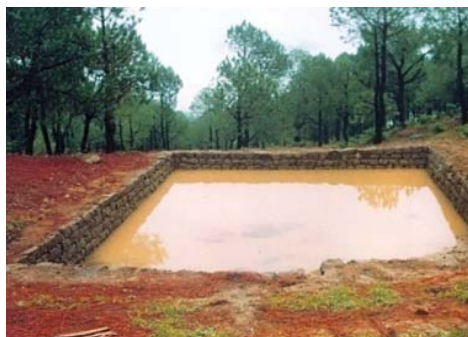
Water harvesting structure constructed
