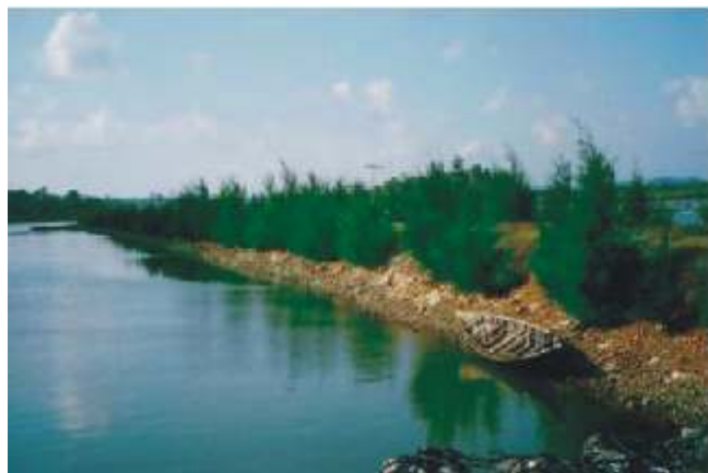
Embankment Plantation at Sippighat (South Andaman)
