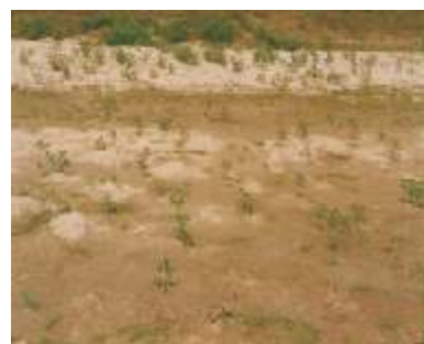
Bunds and Mating with treated Bamboo and Ipomoea plantation for soil stabilization
