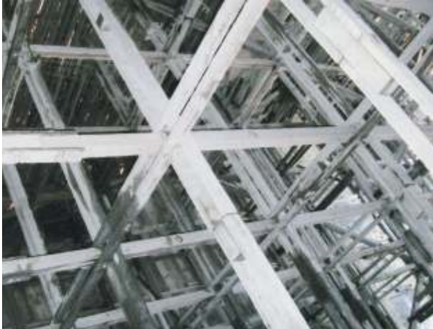
Timber structure inside the cooling tower
