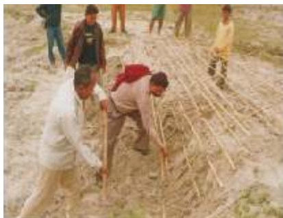
Bunds and Mating with treated Bamboo and Ipomoea plantation for soil stabilization
