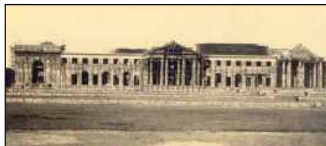
West Block of FRI Main Building under construction
