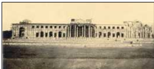
East Block of FRI Main Building under construction
