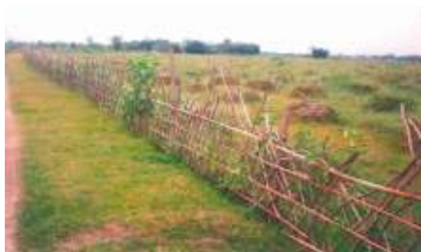
Fencing of site with treated bamboo
