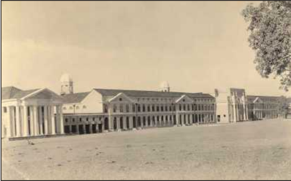
Backside view of the FRI Main Building
