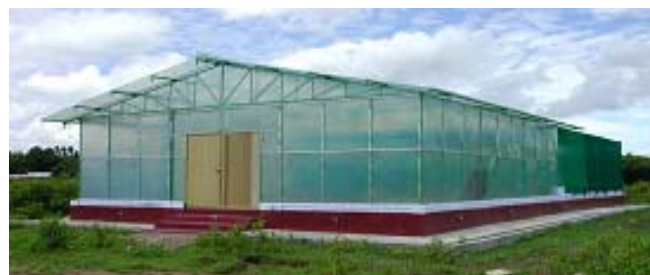
Shade cum poly house constructed under MoEF funded project for development of botanical garden at RFRI
