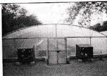
Renovated Polyhouse at Hi-Tech nursery Bikaner
