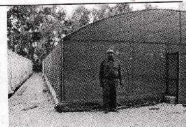
Agronet house after renovation at VVK Satellite nursery, Mohangarh
