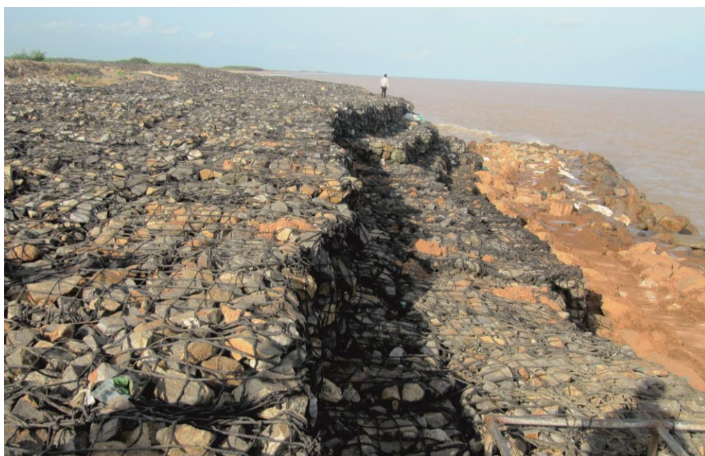
Figure 3: Erosion protection along Pentha coast, Odisha
