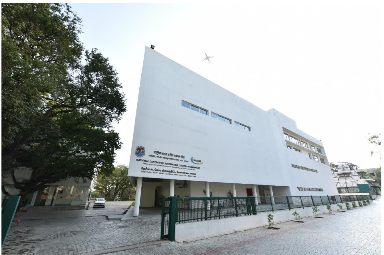
Picture1: Front-view of NCSCM Building
