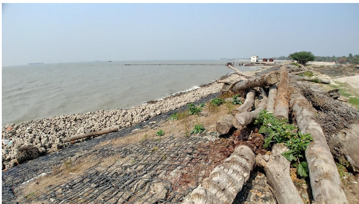
Photo 10: Erosion control measures at Sagar Island
